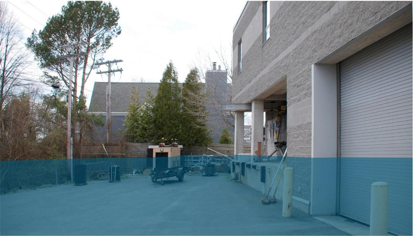
*WWTP Looking West Past the Process Building Depicting Stillwater Flood Elevation BFE + 5-FT*
