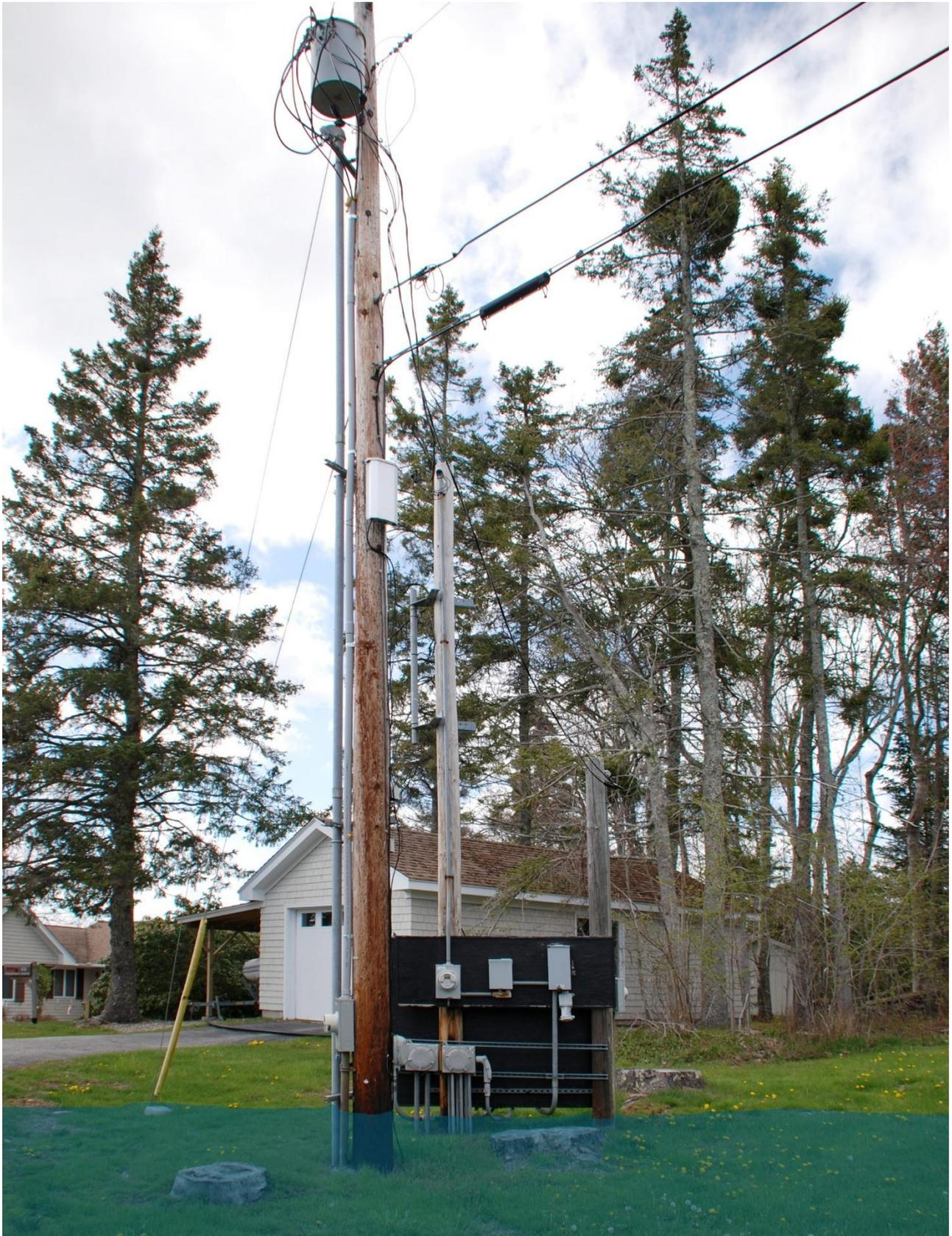
*PS #13 Electrical Service and Controls Depicting Stillwater Flood Elevation BFE + 6-FT*
