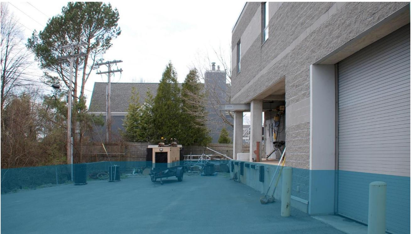
*WWTP Looking West Past the Process Building Depicting Stillwater Flood Elevation BFE + 4-FT*
