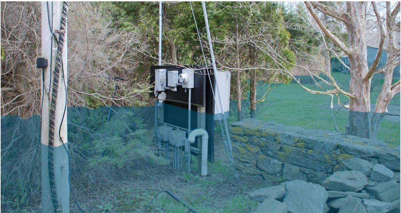
*PS #12 Electric / Control Panel Looking South Depicting Stillwater Flood Elevation BFE + 6-FT*
