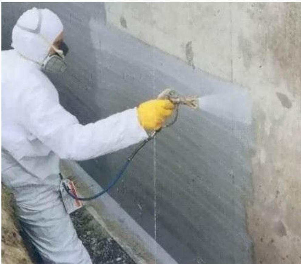
*Example of Spray Coat Waterproofing of Concrete Structure (source from internet)*
