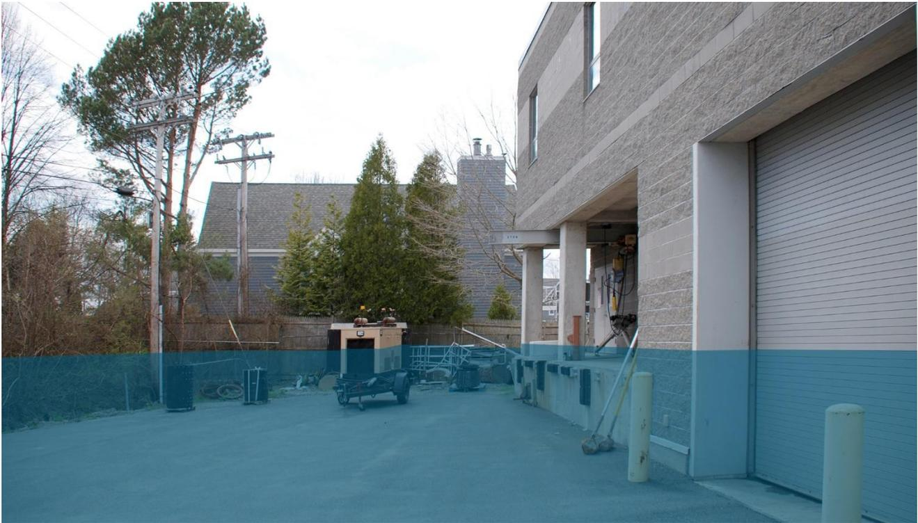
*WWTP Looking West Past the Process Building Depicting Stillwater Flood Elevation BFE + 6-FT*
