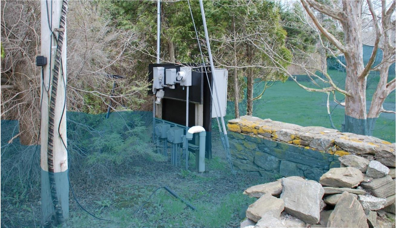
*PS #12 Electric / Control Panel Looking South Depicting Stillwater Flood Elevation BFE + 5-FT*
